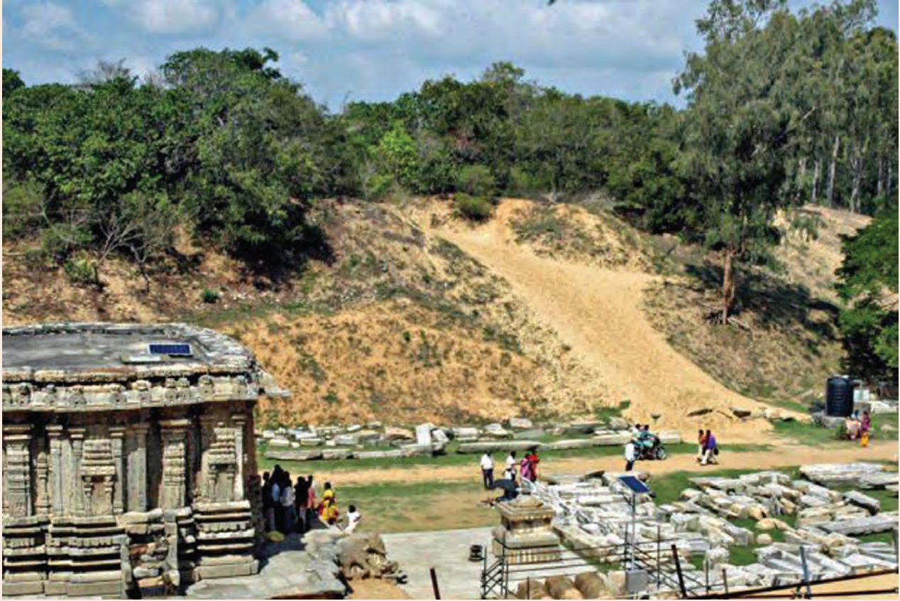
Renovation at Talakadu, T.N.Pura Taluk, Mysuru Dist.
